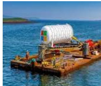
2018: immersed data centre demonstrator
